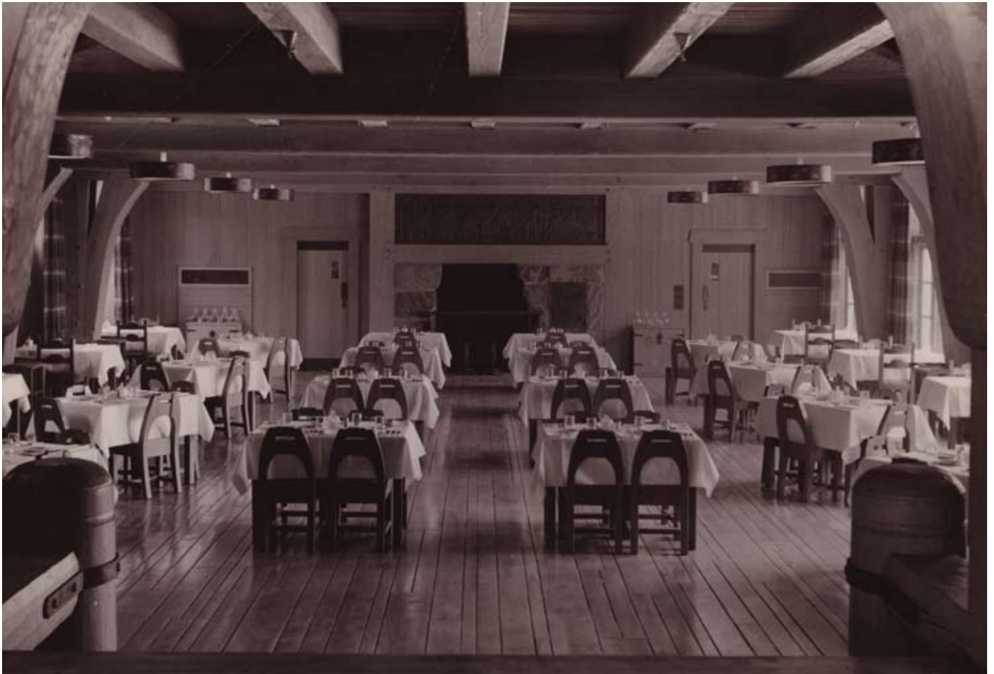
Timberline Lodge, Dining Room, Mt. Hood, Oregon, Friends of Timberline Archives
